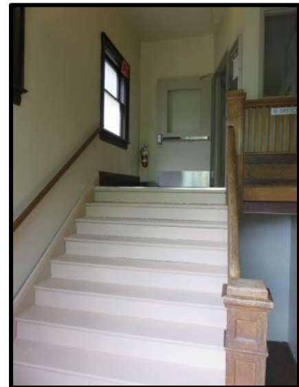
Walls and stairs with a fresh coat of paint!
