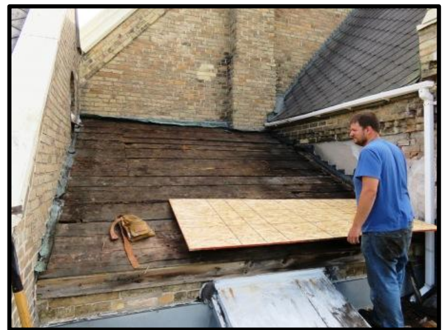
Mr. Howard repairing the organ chamber roof.
